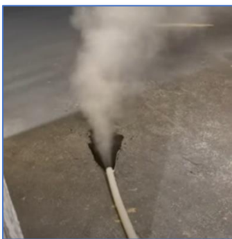
Figure 24 – Illustration of Steam and Liquid Safely Coming Out of Venting Hose
